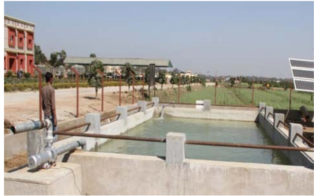
b) Delivery unit lifting water out of storage tank for irrigation at high head
