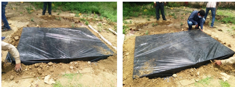
Water tank covered with plastic sheet during mid July 2020
