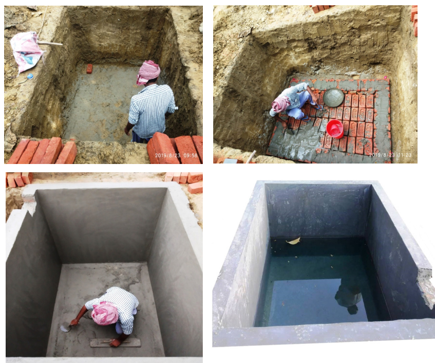
Fig. 1. Construction of brick lined rain water storage structure
